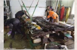
Removal of a timber with the crane
